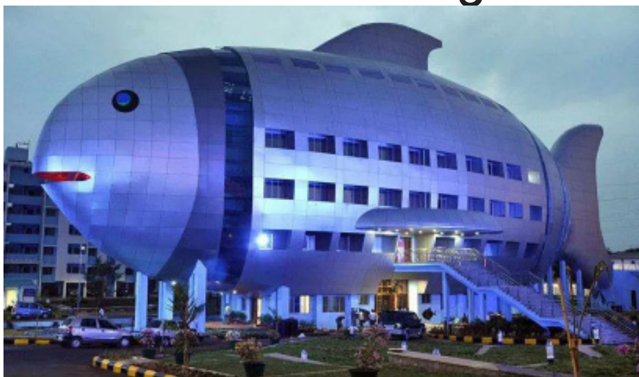
Hyderabad: Adding another feather to the cap, the National Fisheries Development Board (NFDB) building in Hyderabad, colloquially known as 'The Fish Building', has
