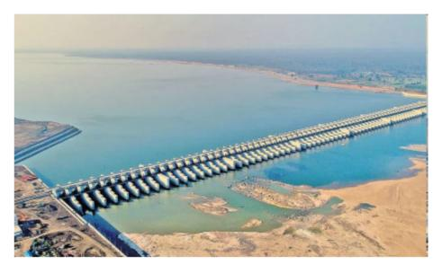
Medigadda to manage the high-pressure force released from the gates of the barrage during flood. Extension of the apron of the barrage by at least another 45 metres was recommended. A sampling study conducted by L&T revealed that the non-construction of a tail pond below the Medigadda barrage has led to significant soil erosion and the formation of large potholes, which have gradually caused sand to slide under the foundations of the barrage. To address these issues, the Irri-
